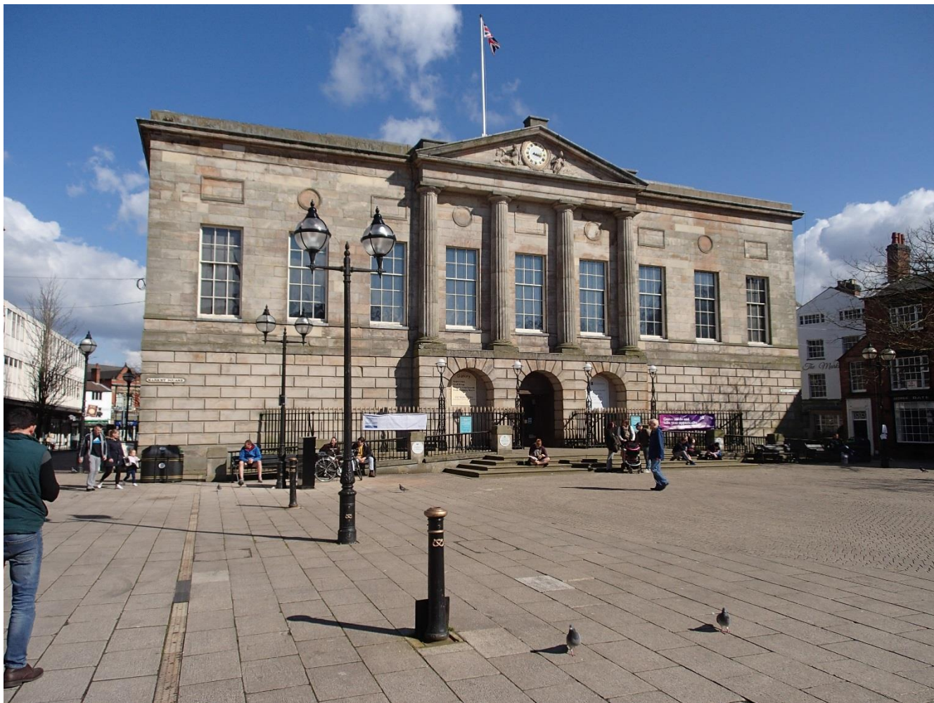
Shire Hall, Stafford. Photo: John Dearing
