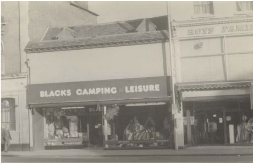
Left: a very strange building, 62 St Mary's Butts. It used to have two sash windows on the first floor, but these were removed in the 20 th century. It is evident this was refronted because of the irregular roofline and dormers. Demolished at some time in the last 40 years.
