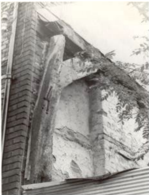
Left: 90 London Street, 1973. Here we can see the brick front to Church Street, and behind it, timber-framing. After this was taken, number 90's facade was preserved while the timber-framed section was demolished, a similar arrangement to the fate of nos. 49-53 London Street.
