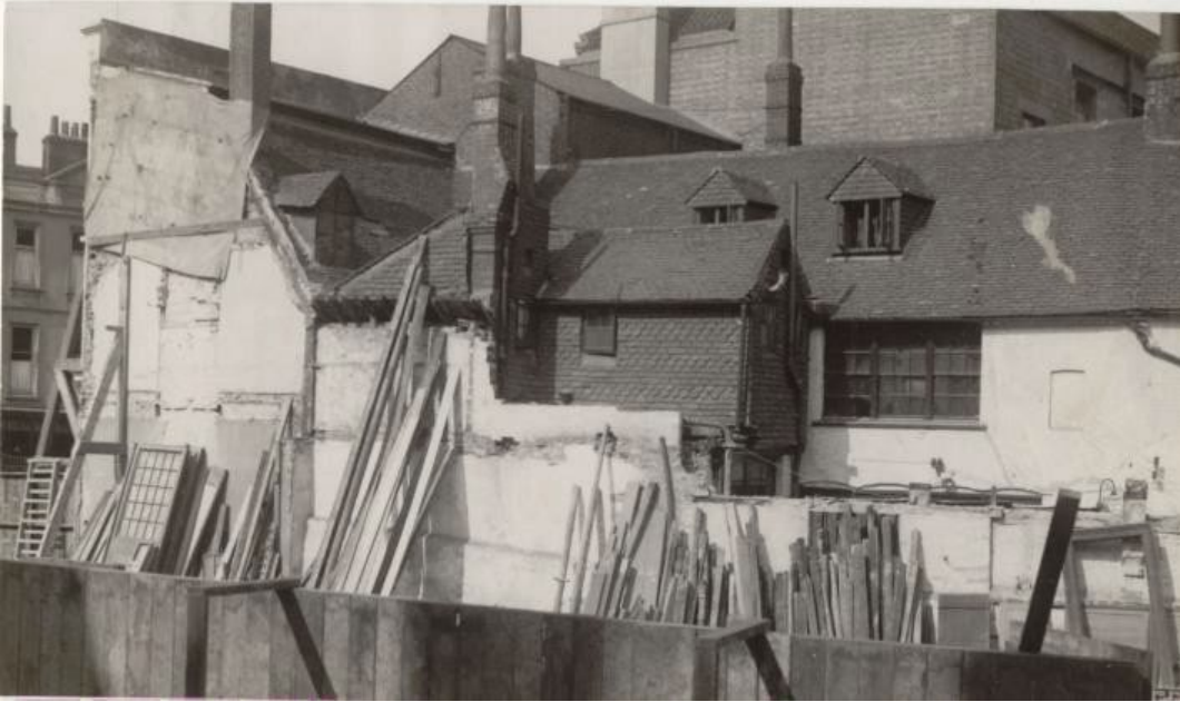
Left: 5-6 Friar Street, The Wheatsheaf, 1929. This timber-framed range was exposed when the corner site adjoining was demolished to make way for Somerset House. It was demolished in about 1960.
