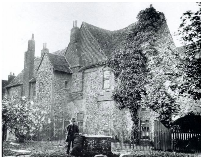
Left: The Hospitium before restoration, seen in the 1880s
