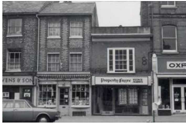
Left: 43 London Street, 17 th century and demolished in the last few years. On the right is 105 London Street.
