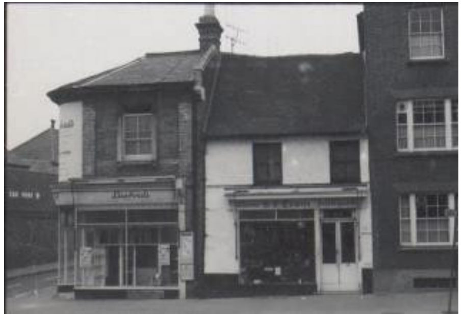
Right: the white building in the middle was 69 London Street, another photograph of which appears earlier on. Its facade was 18 th century, fronting a timber-framed house. We know it was refronted, as when its timber-framed internal structure collapsed (possibly due to neglect) the frontage did not fall with it, meaning it was not connected to the rest of the house.
