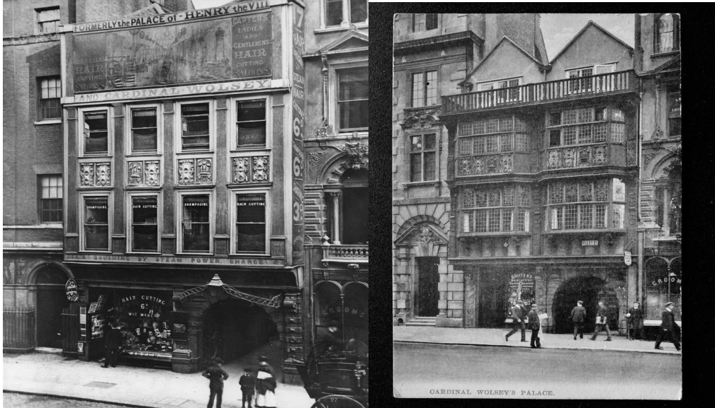
Inner Temple Gatehouse. Left: before removal of façade; Right: after
